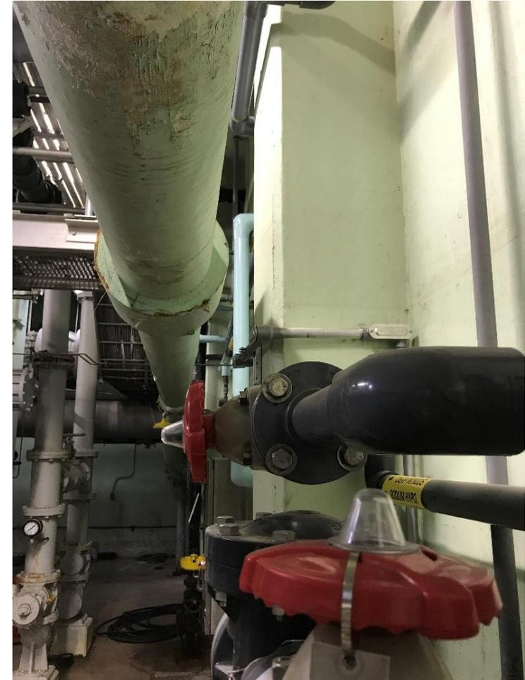
The pumps and controls to be along this wall with discharge piping heading south through tunnel
