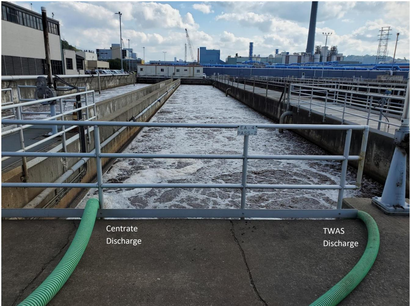
**Figure 4.** Centrate and TWAS hoses discharging into EA-4 Pass-2.
