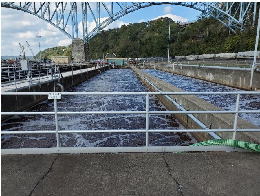
**Figure 4.** WAS feed hose pulling out of EA-4 Pass-1.
