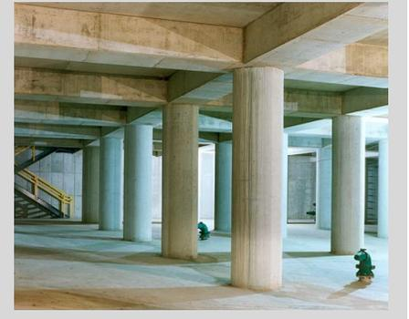
The basin storage facility above, located in Van Buren Township, Michigan, is an example of one of the types of control technologies being evaluated to control overflows in the LOGR Basin. This 1.3-MG storage basin is used to balance sewage flows between available capacities in three regional sewer systems. It is covered by earth and features green storm water management practices including a bioswale and storm water reuse to flush the basin after use.
