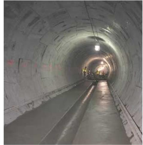
The photograph shown above is a typical underground storage tunnel. Identified as a potential Wet Weather Control Alternative, storage is the process of controlling the flow rate to a wastewater treatment system by temporarily storing the overflow volume and discharging it to the treatment plant at a controlled rate.
