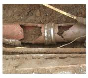
capacity, and cracked and deteriorating pipes allow infiltration of additional rain and snow melt. Overgrown tree roots in the pipes can inhibit flow. In addition, many households have improperly connected downspouts or sump pumps which force stormwater into sewer lines designed to carry only sewage.
