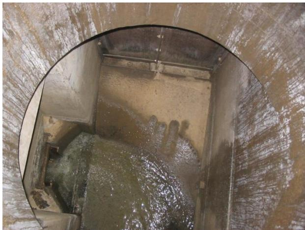
**Figure 3-4: Interior view of an ALCOSAN regulator structure diverting flow for treatment**
