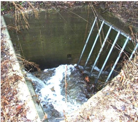
**Figure 3-8: A creek along Spring Garden Avenue is culverted and becomes the Spring Garden combined trunk sewer serving Reserve Township and the City of Pittsburgh.**
