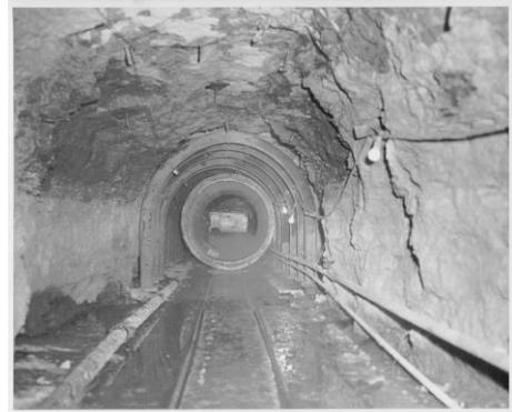
**Figure 3-2: Construction of an ALCOSAN deep tunnel interceptor sewer**
