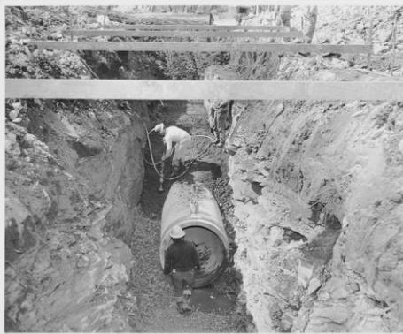
**Figure 3-3: Construction of an ALCOSAN shallow-cut interceptor sewer**
