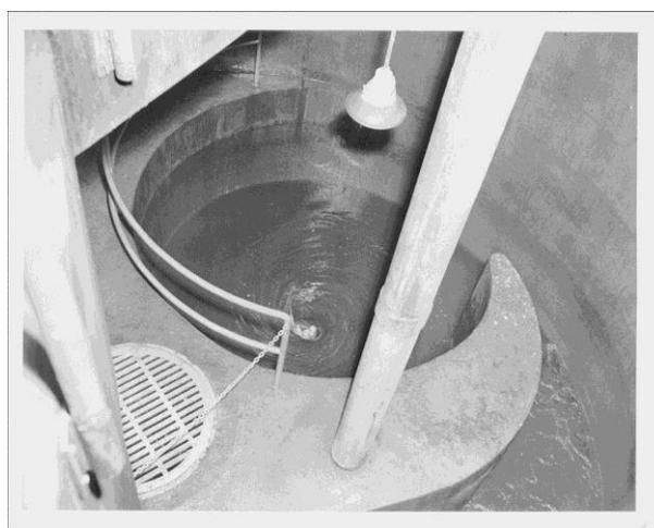
**Figure 4-14: Typical example of a vortex drop-shaft used to convey flow to the deep tunnel system**
