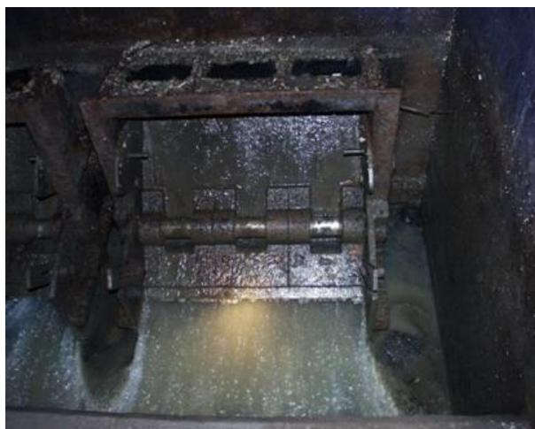
**Figure 4-13: Typical example of a variable-orifice tipping gate used to regulate wastewater flow**
