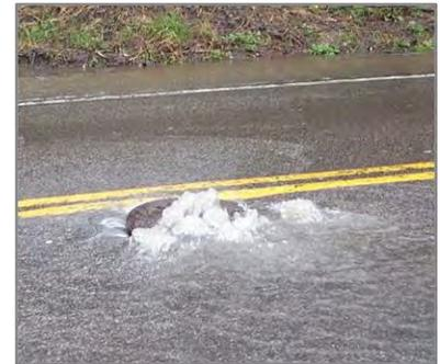
*Figure 6-8: Sanitary Sewer Overflow Caused by Excessive Inflow and Infiltration*
