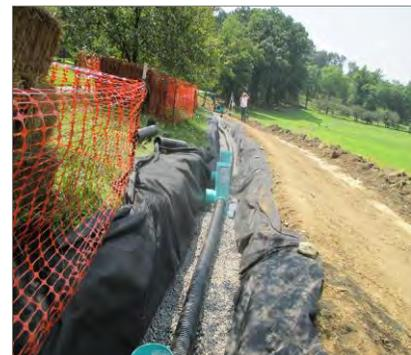
*Figure 6-9: Infiltration trenches and berms have been installed to reduce hillside erosion, converting lawns to meadows, and vegetative buffers in Pittsburgh’s Schenley Park.*
