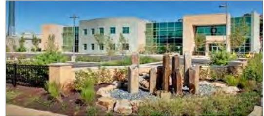
*Figure 6-10: ALCOSAN's CS&T Building parking lot uses a rain garden and bio-swale to capture and infiltrate stormwater*
