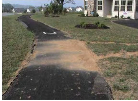
**Figure 2-13. Material Storage and Sediment on Permeable Pavements**
