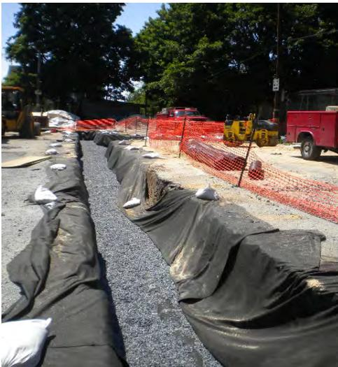
**Figure 2-5. Geotextile Installation**
