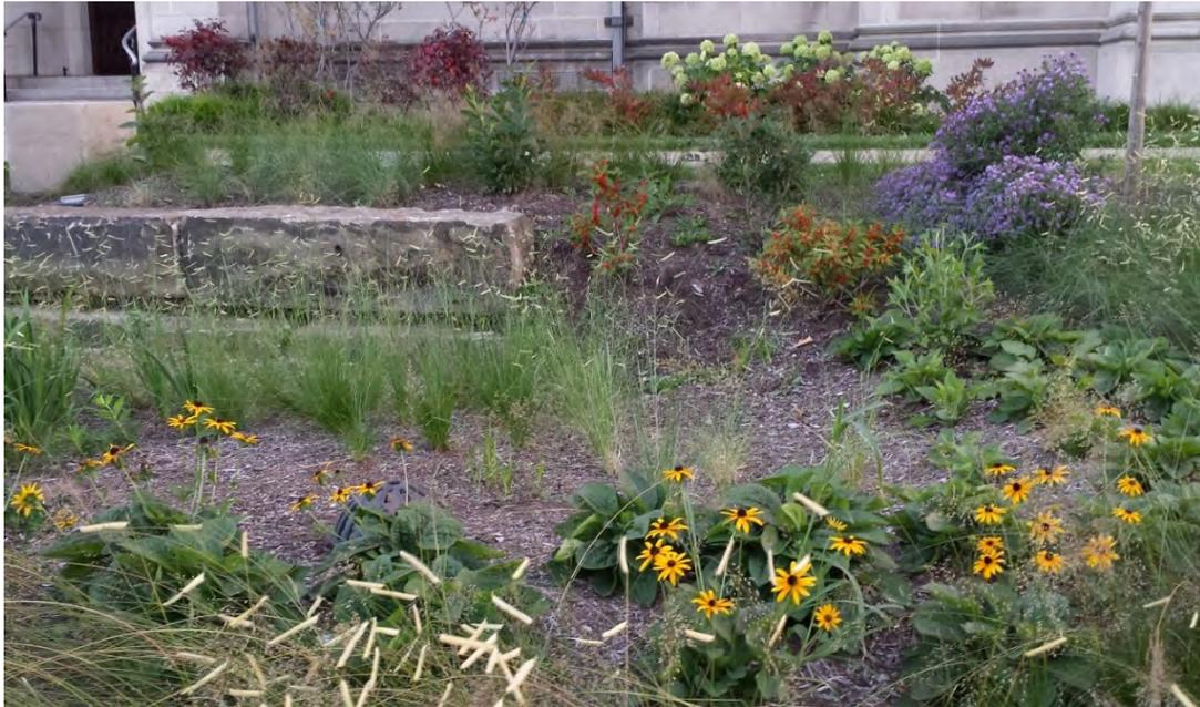
**Figure 2-1. Bioretention Basin**
