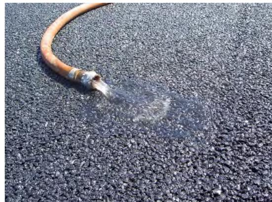
**Figure 2-11. Porous Asphalt**
