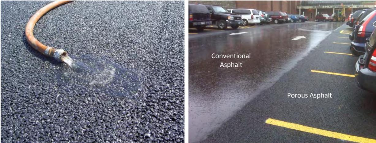
Figure 2-12. Porous Asphalt Surfaces
