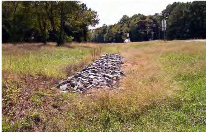
Figure 2-10. Surface Flow Infiltration Trench
