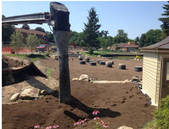
**Figure 2-6. Soil Slinger Truck**
