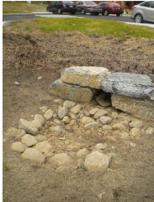
**Figure 2-7. Sediment in Bioretention Area**
