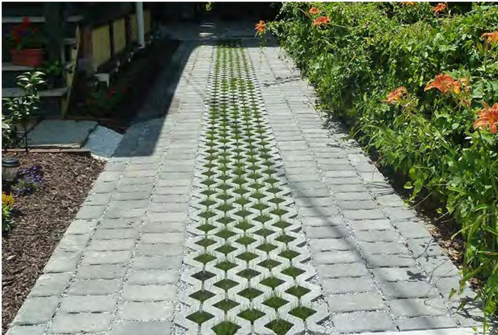
**Figure 2-15. Open Grid Pavers**
