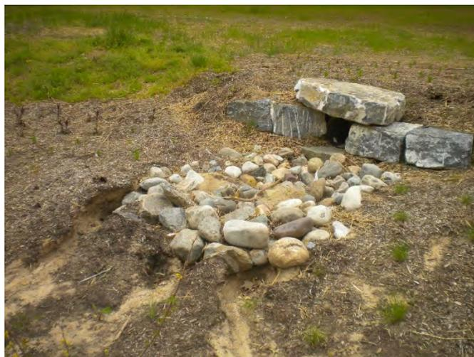
**Figure 2-3. Erosion in Bioretention Area**
