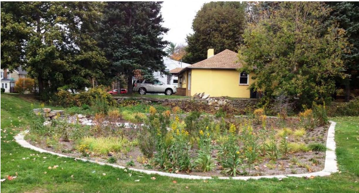
**Figure 2-16. Bioretention Area**
