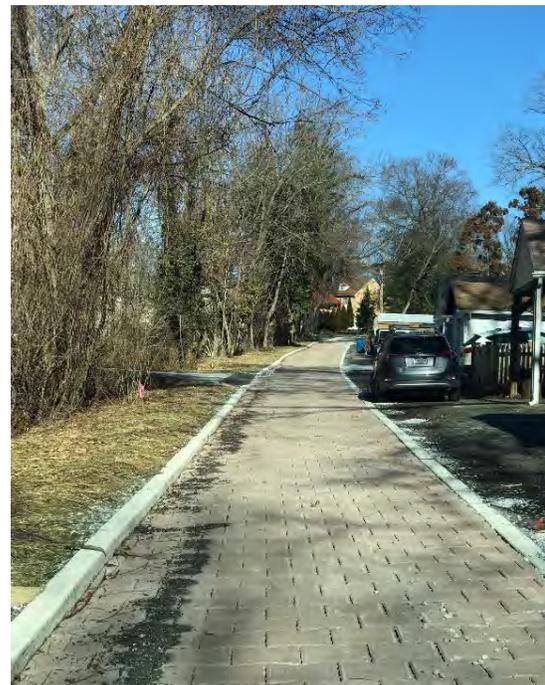
**Figure 2-14. Excess Gravel on Permeable Pavers**
