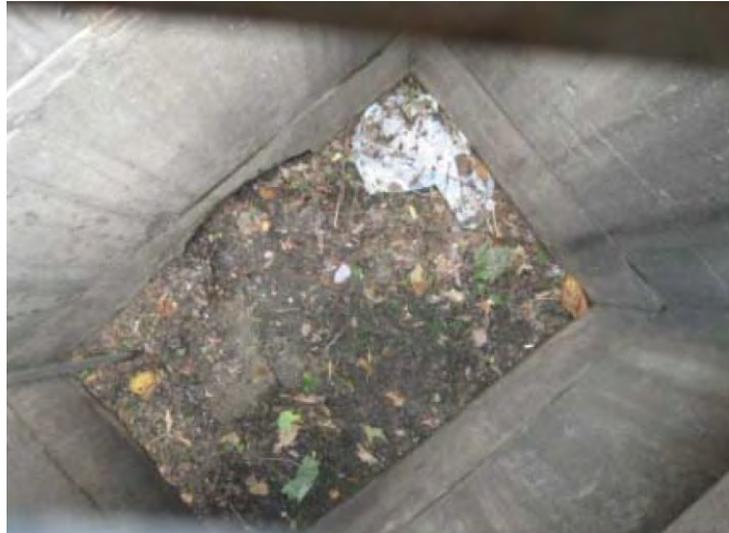
**Figure 2-10. Sediment and Debris Clogging of Inlet**
