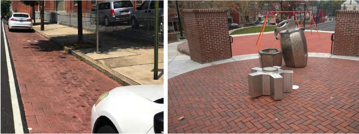
**Figure 2-14. Permeable Pavers**
