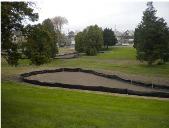
**Figure 2-3. Silt Fence Around GSI**
