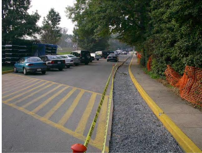
**Figure 2-8. Infiltration Trench**
