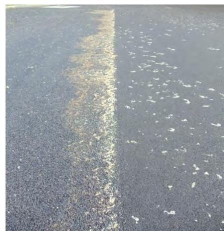
**Figure 2-1. Debris on Porous Asphalt**
