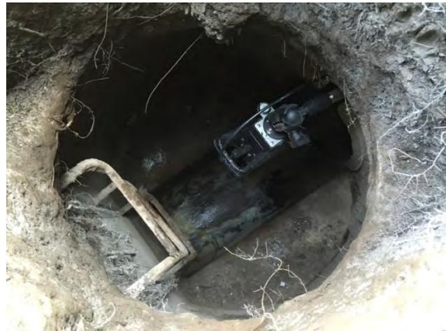
Figure 2-9. Area-Velocity Meter Installation Setup in Sewer (Flow-Tronic)
