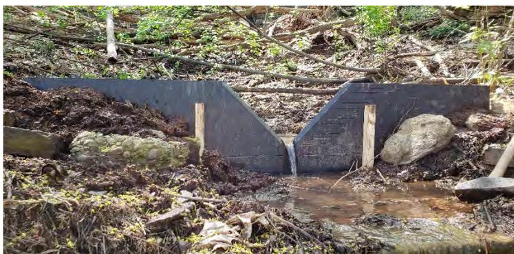
Figure 2-5. V-notch Weir (PWSA)
