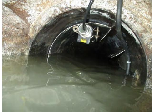
Figure 2-8. Area Velocity Meter Installation Setup in Sewer (RJN Group)
