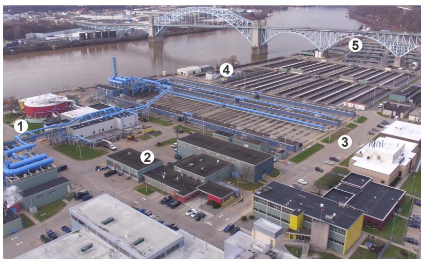
*Planned upgrades include a new pump station (1), expanded headworks (2), additional primary tanks (3), and a new wet weather bypass and disinfection system (4) required to expand maximum wet weather flow to 600 MGD. In addition, secondary treatment will be expanded to 295 MGD with a new disinfection system and a relocated outfall (5)*
